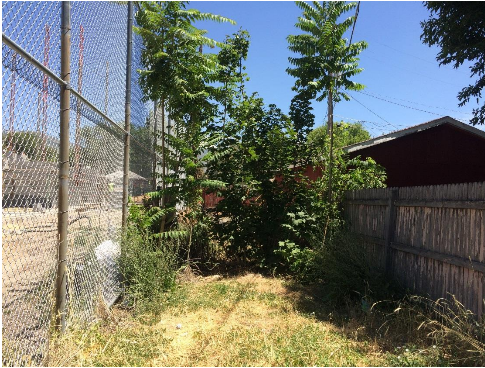
Encroachment into the alley behind the property located at 269 East Hampton Avenue.
